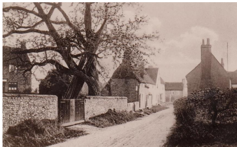
View down Free Street to the Wheatsheaf on the left before the end bay extension and the house opposite was demolished (Photographer probably T. Duffett) BW150031
