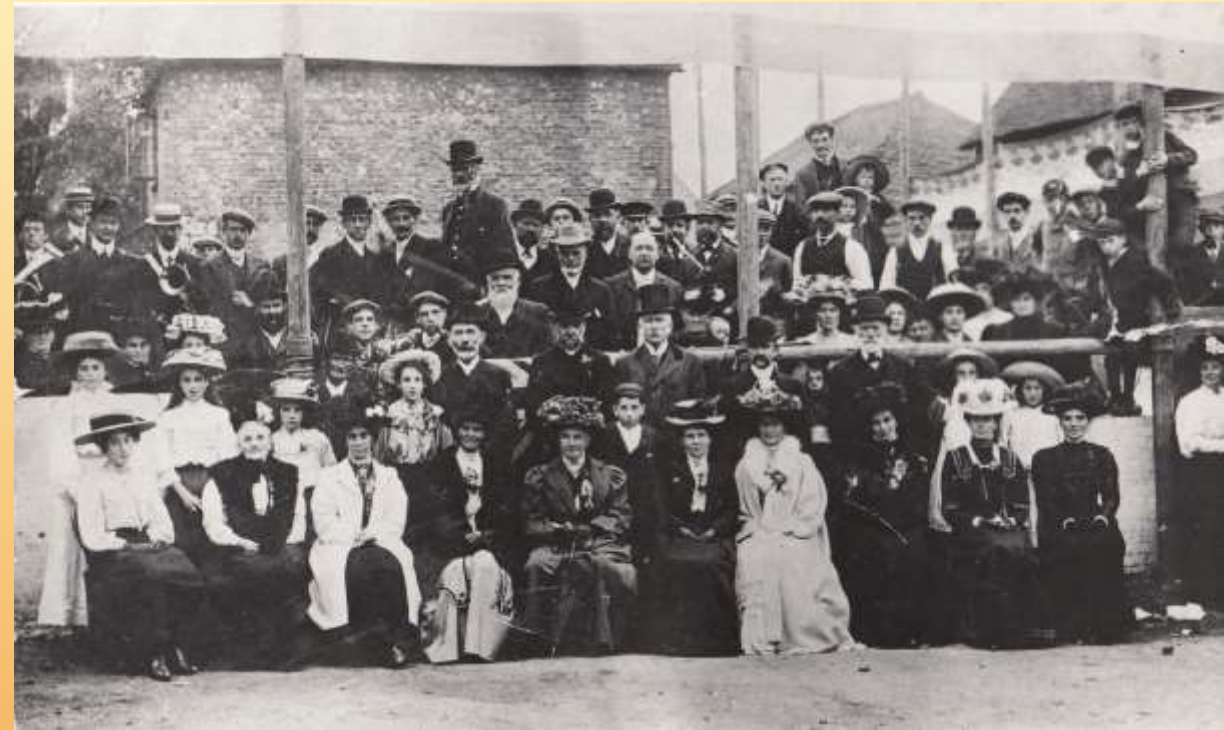
1909 St Paul's Methodist Church Foundation Stone laying celebration at Basingwell Street Photo: Unknown
