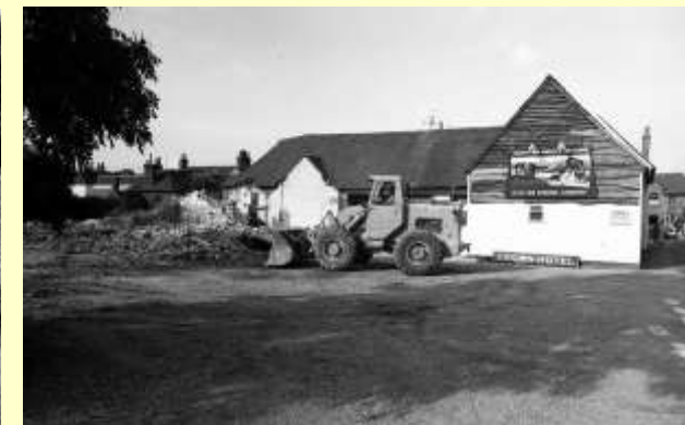
Rear of Crown Inn with stables being demolished, 13 September 1968 (John Bosworth)
