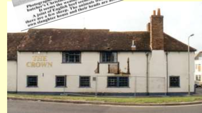
The Crown with original beams exposed, 1997 (John Bosworth)
