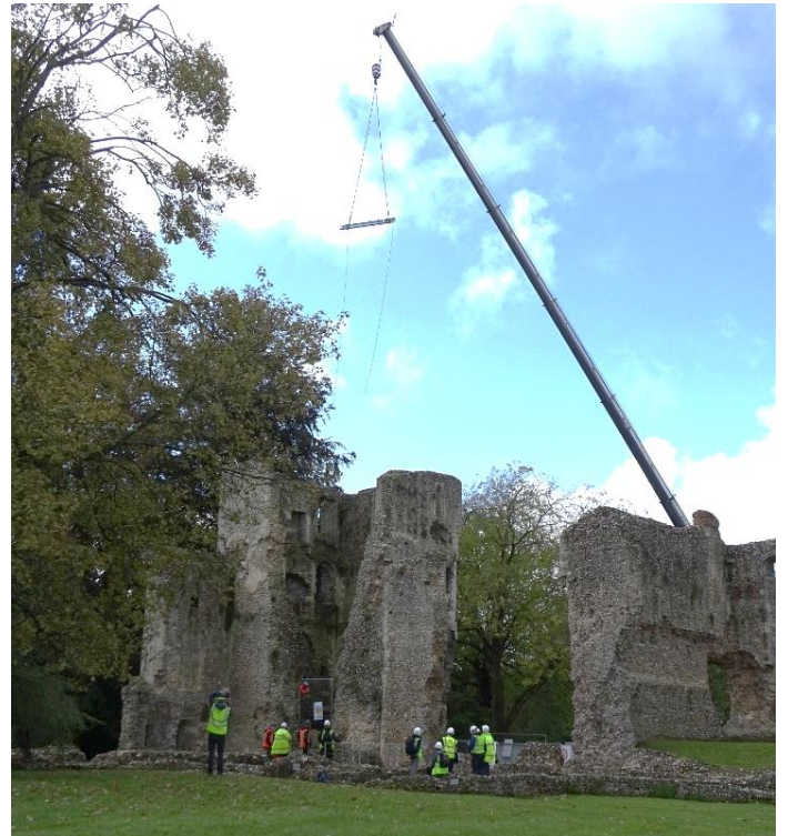
Part of the structure being craned in...
